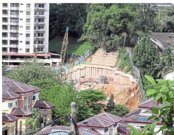
Holding back: A developer working on reinforcing a hill slope to prevent landslides along Persiaran Syed Putra, Kuala Lumpur. The repairs follow growing concerns about slope stability. — ART CHEN/The Star
